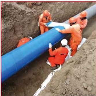
Viscotaq Viscowrap™ In Wrap Viscotaq™ Outer Wrap (PVC, PE, HDPE o Glass Wrap, se richiesto)
